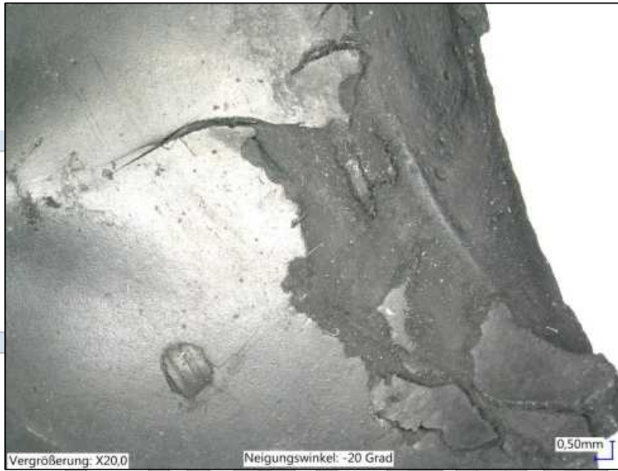
Figure 1: EPDM-seal destroyed by disinfectant
