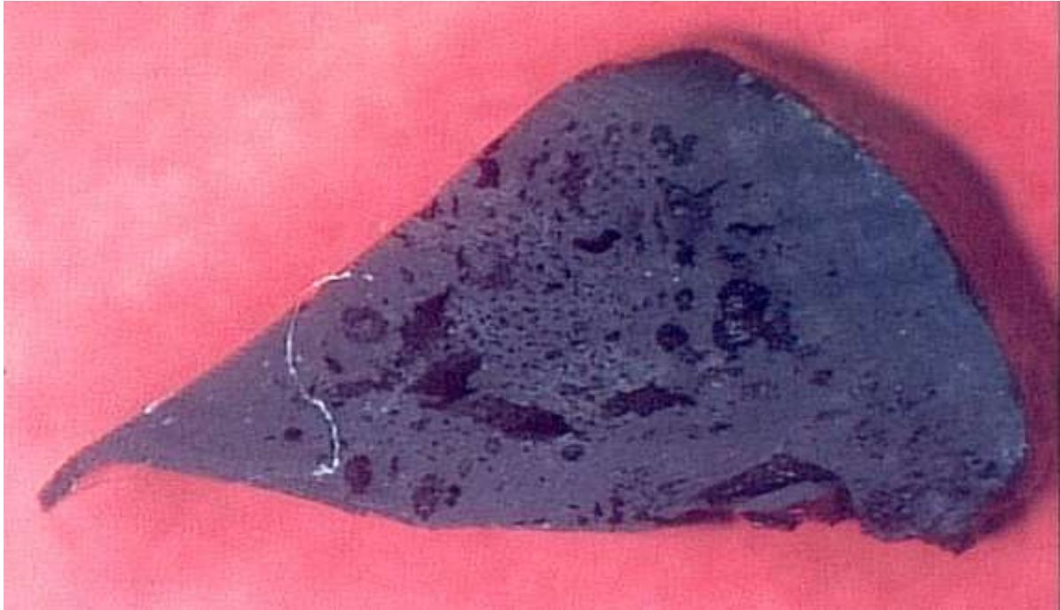
Figure 3: FKM O-ring (Aflas) after a service of about 5 years in an armature of a district heating network at hot water temperatures up to 170°C (triangular groove)
