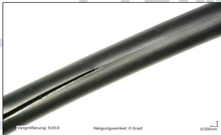
Fig. 7: Assembly-related crack due to the impact of a sharp edge in the installation space
