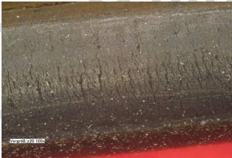
Fig. 22: Cracks due to aging due to heat and oxygen under slight elongation can be seen on the contact surface of an O-ring
